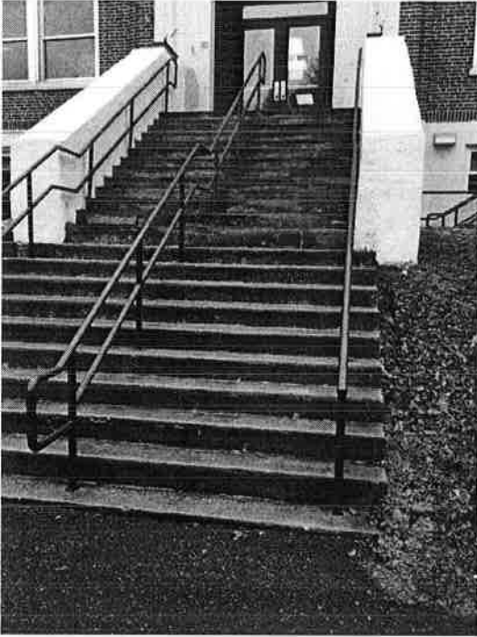
Main entry stairs and rails
