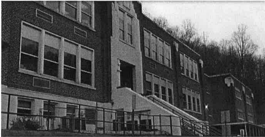
Front of original building and 1967 addition
