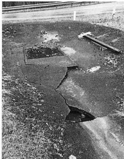
Storm Water Basin
