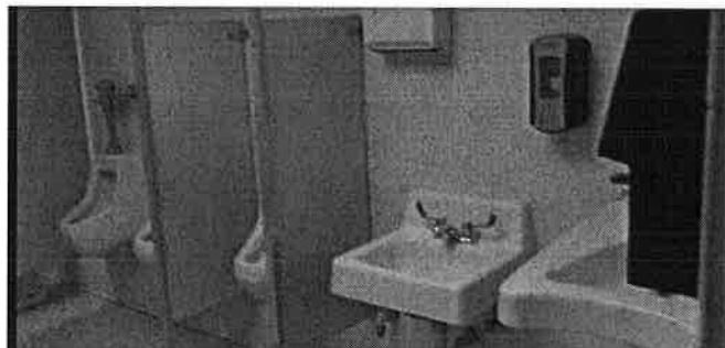
Boys restroom in classroom area
