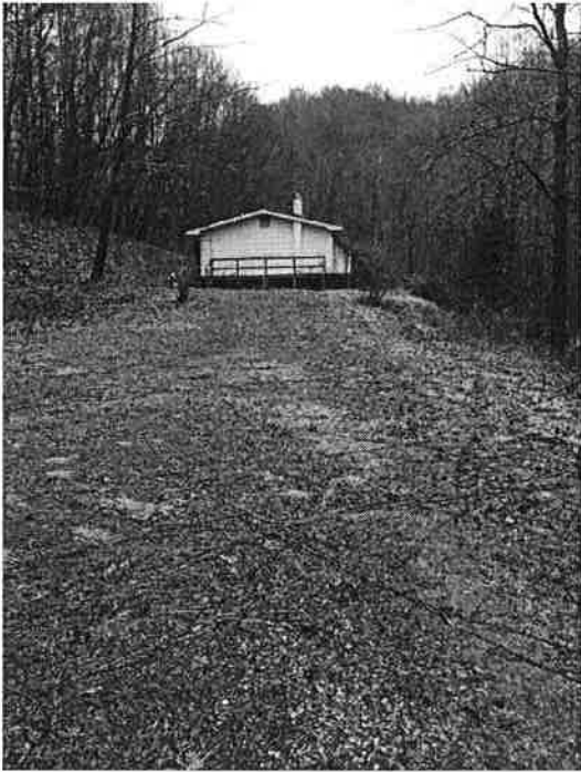
Janitors house and gravel drive
