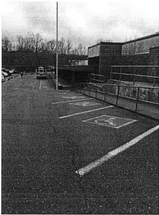
Bus Loading Area
