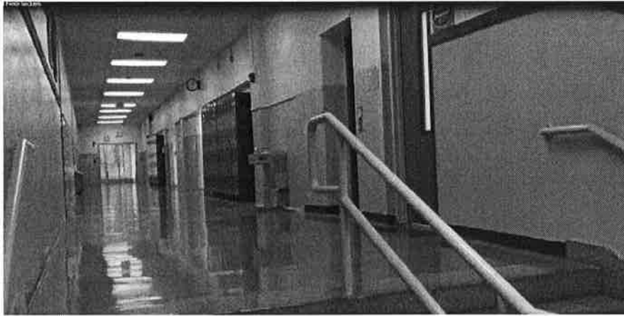
Upper floor classroom corridor
